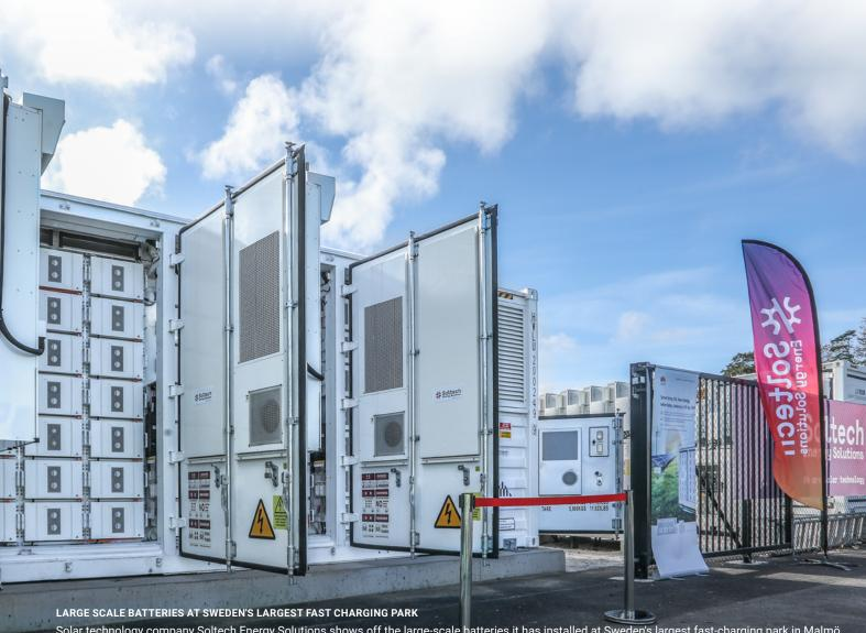
Solar technology company Soltech Energy Solutions shows off the large-scale batteries it has installed at Sweden's largest fast-charging park in Malmö during an event in October. The park is equipped with 2 MW batteries that both relieve the grid and ensure high capacity in the fast chargers. The park will accommodate both heavy electric transport vehicles and private electric cars.
